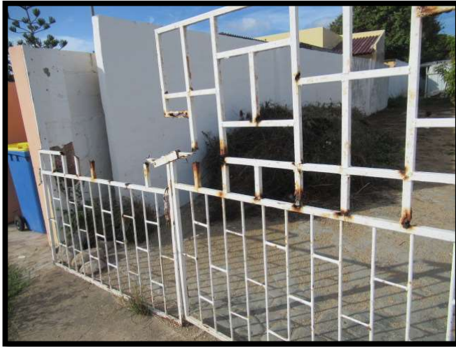
Condition of the steel fence gates and railing at Pampunastraat 15-G.
