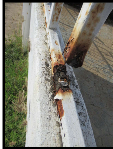
Condition of the steel fence gates and railing at Pampunastraat 15-G.
