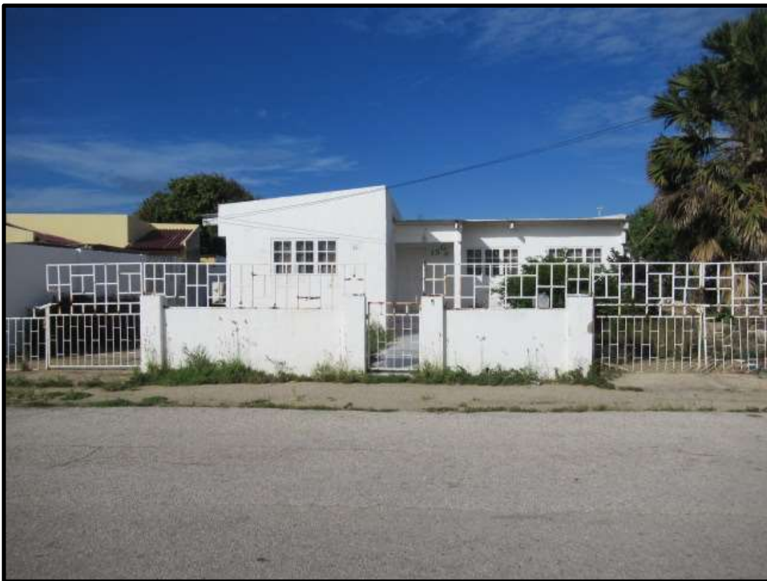
Front view of the concrete block house at Pampunastraat 15-G.
