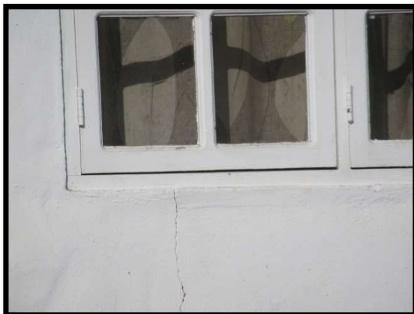
Crack in exterior wall at Pampunastraat 15-G.
